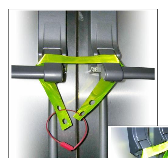
Security seal and sash system for push bar type emergency exits.
